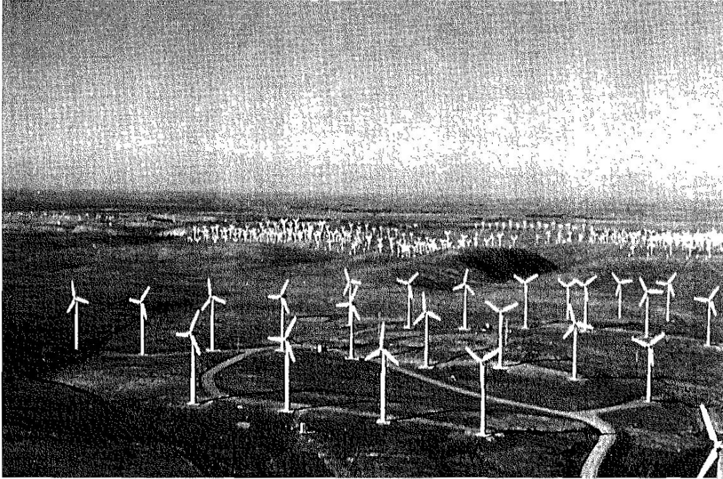
Figure 12.24: Wind farm located in Altamont Pass, near Livermore, CA. Maximum power output is 5\text{ MW} at a wind speed of 15\text{ mph} . Courtesy U.S. Department of Energy.
